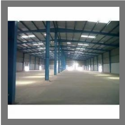
Aluminum Roofing Shed
