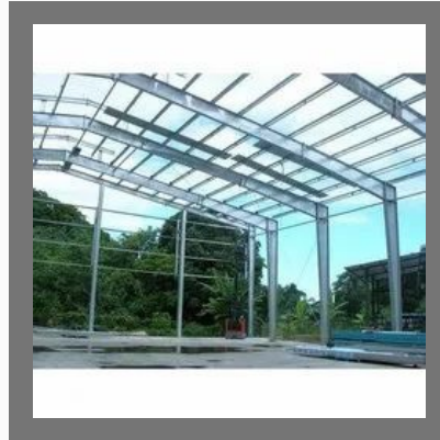
Steel Prefabricated Shed
