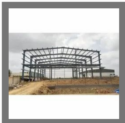
Steel Roofing Structure
