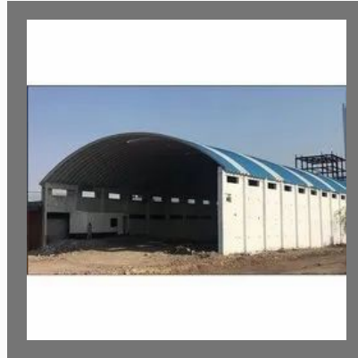
MS Industrial Roofing Shed
