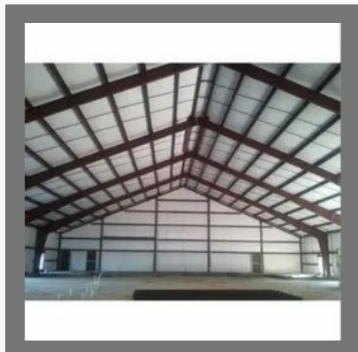
Factory Roofing Shed
