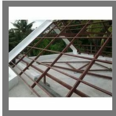
Mild Steel Roofing Structure
