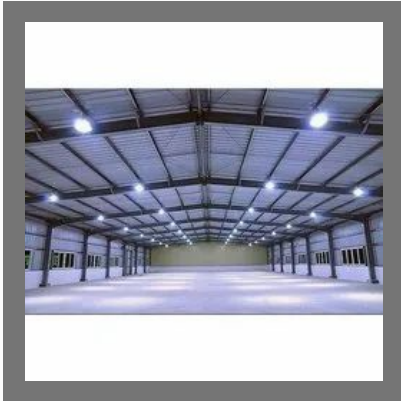
Prefabricated Steel Roofing Structure
