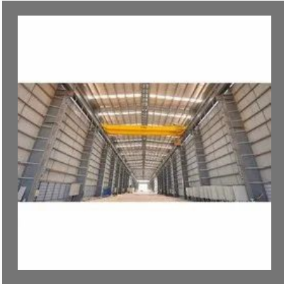
MS Prefabricated Shed
