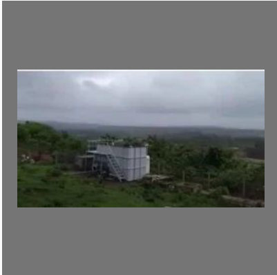
Sewage Treatment Plant
