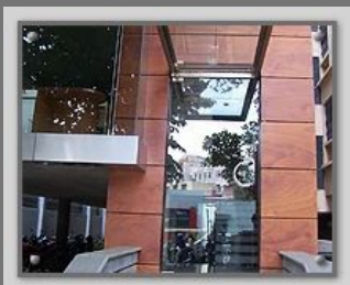
Window & Door System
