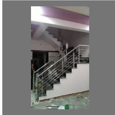
Steel Stairs Railing
