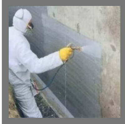
Anti Termite Treatment
