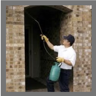
Pre Construction Anti Termite Treatment
