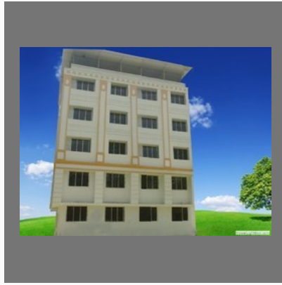
Sri Krishna School Building Construction Project
