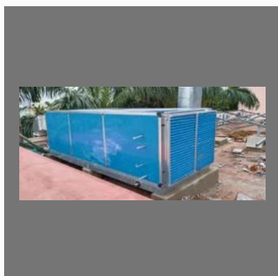
Voltas Central Ac repair and service
