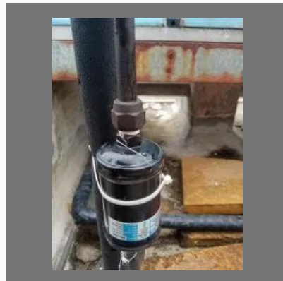
AC Gas Pipe Line Installation Service
