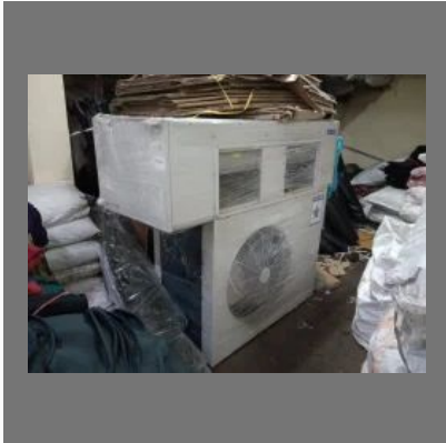
Split Ac Repair Services
