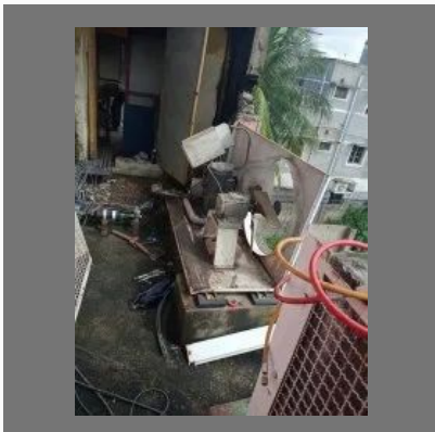
Ductable Ac Installation Services
