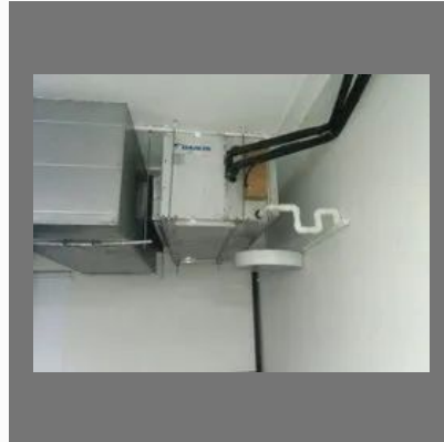
Package AC Installation Services
