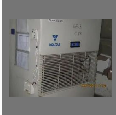
PACKAGE AC UNIT REPAIR AND SERVICE
