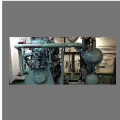
Marine AC Maintenance service
