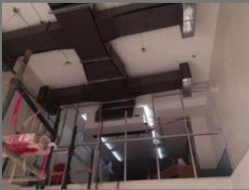
Shopping Complex AC Unit Repairing and service
