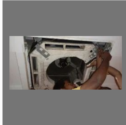
Cassette AC Repair and service
