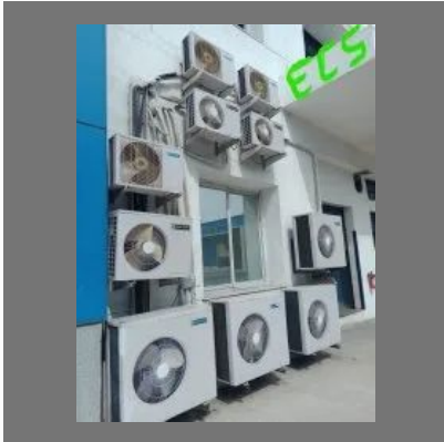
Daikin Ductable Ac Repairing Services
