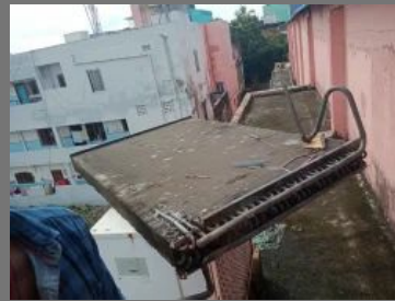
Ac Condenser Coil Repair Service
