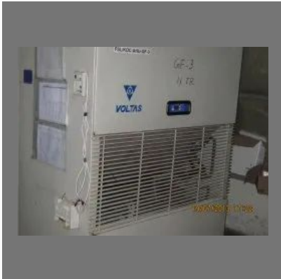
Package Ac Repair and Service
