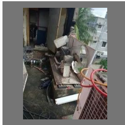
Ductable Ac Installation Services
