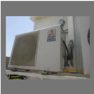
Cassette Ac Repair And Service
