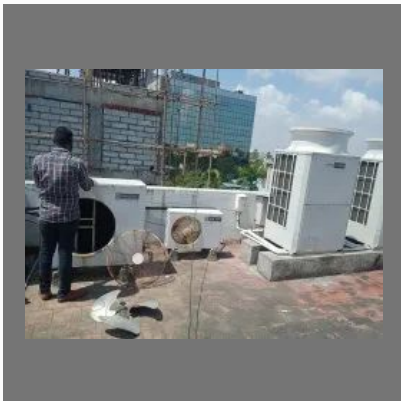
AC Pipe line Gas Leak Work Service
