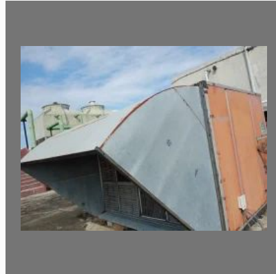
Ac Duct Installation Work service
