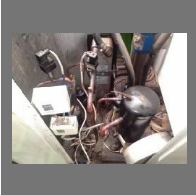
AC Compressor Repair and Service
