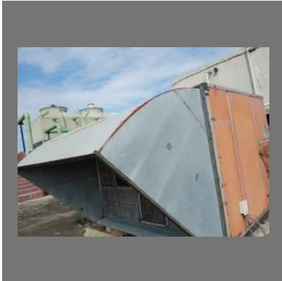
Ac Duct Installation Work service
