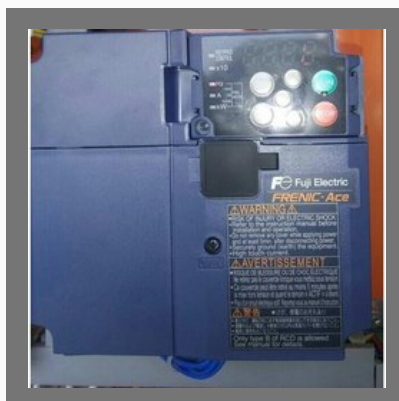
Fuji Elevator VFD
