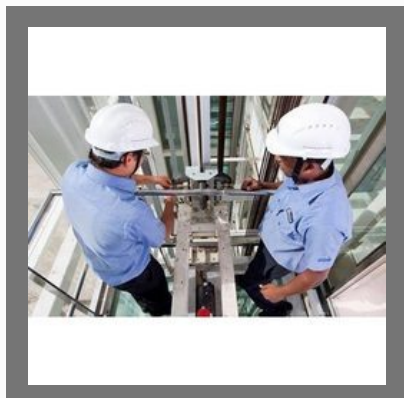
Elevator Repairing Service
