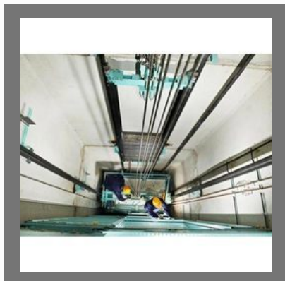
Elevator Commissioning Service
