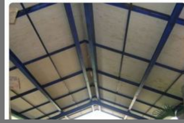
Factory Shed Fabrication
