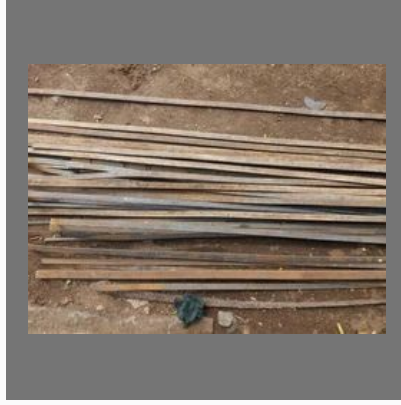
Railing Fabrication Work
