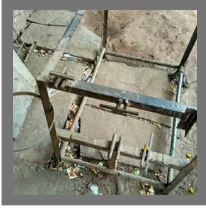
ST Shut Fabrication Work
