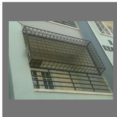
Balcony Railing Fabrication
