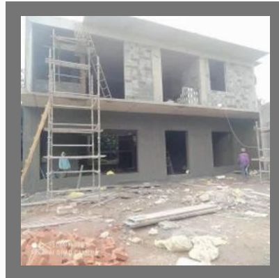
Building Construction Civil Work
