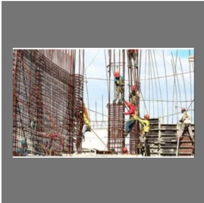
Commercial Building Construction
