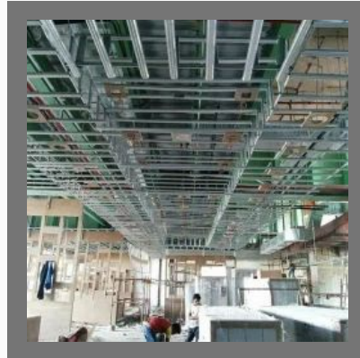
Construction Service & work
