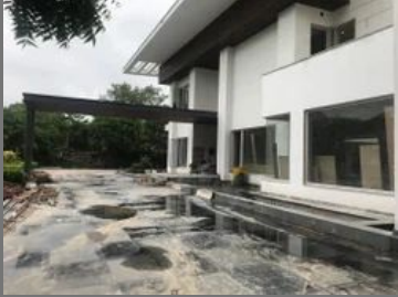
civil construction contractors
