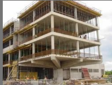
Commercial Construction Service
