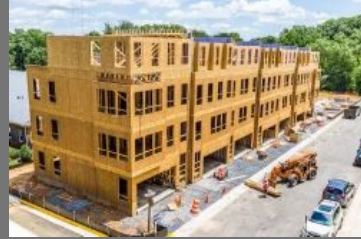
Institutional Construction projects
