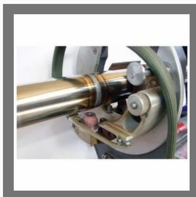
Orbital Welding Work
