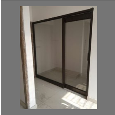
Aluminium Sliding Door Work
