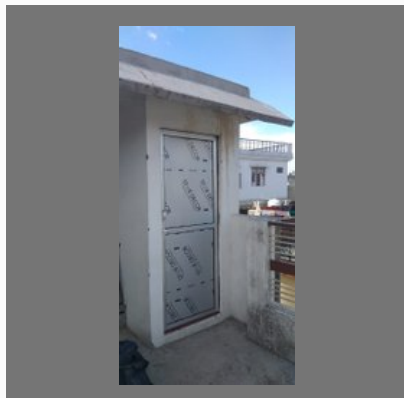
Aluminum Doors Fabrication
