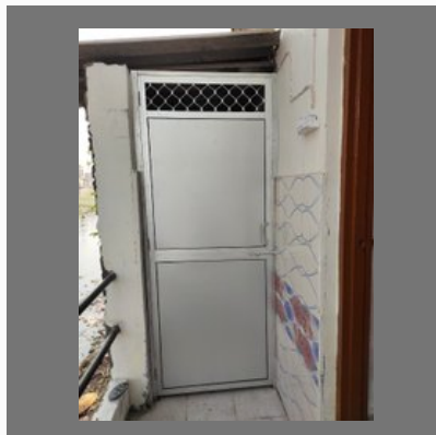
Aluminum Doors Fabrication
