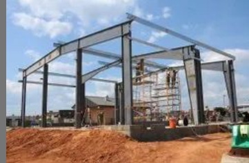
Prefabricated PEB Sheds Building Structure Work
