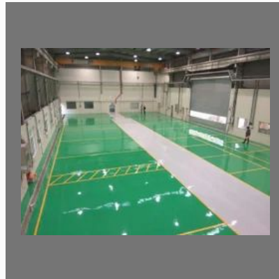
Abrasion Resistant Epoxy Flooring
