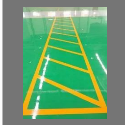
Epoxy Self Leveling
