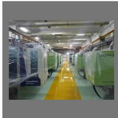
Epoxy Floor Topping
