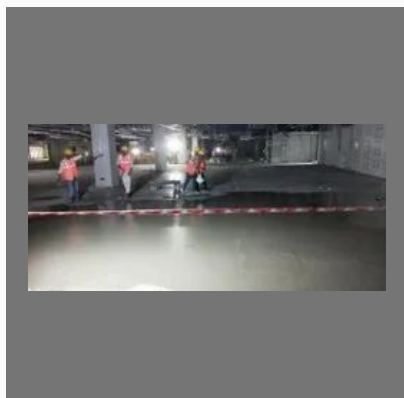
Self Leveling Flooring Service
