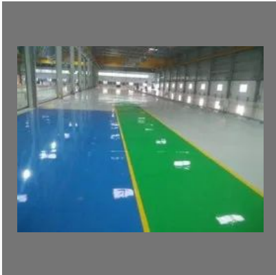
PU Floor Coating Service
