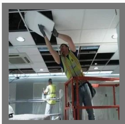
False Ceiling Services
