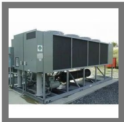
Air Cooled Chiller
