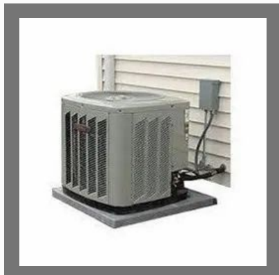
Air Conditioner Condenser
