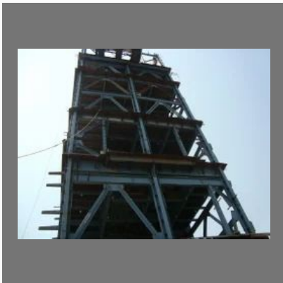
Heavy Structure Fabrication Of Crusher House
