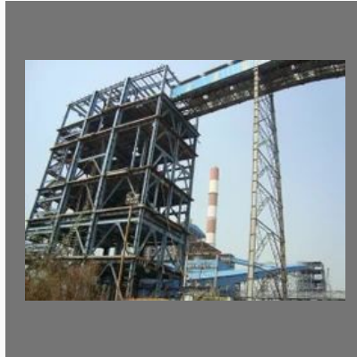
Conveyor Structure Fabrication
