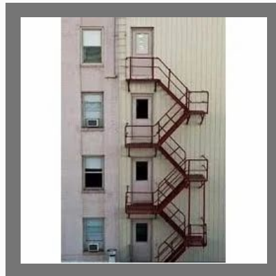
Fire Escape Staircase
