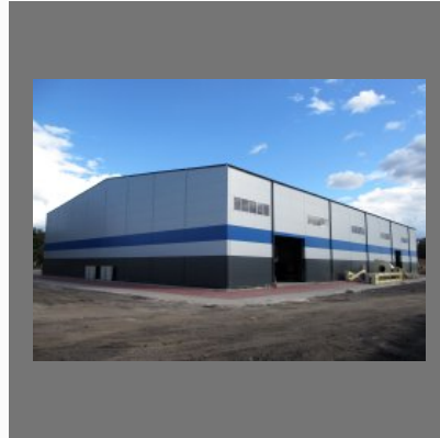
Production Plant Warehouse Construction Services
