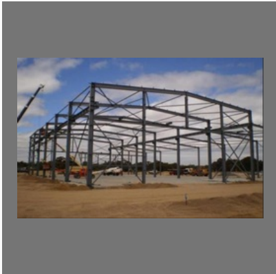
Industrial Building Construction Services
