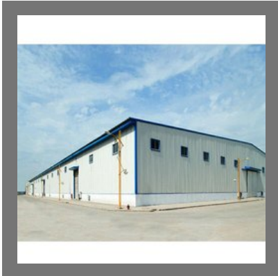
Prefabricated Factory Shed
