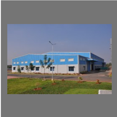
Industrial Building Construction Services
