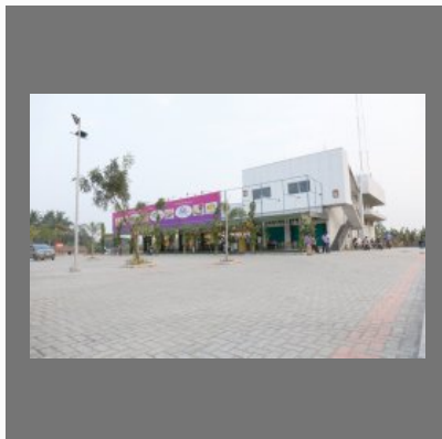
Construction Of Commercial Building
