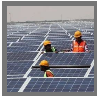
Solar System Installation Service
