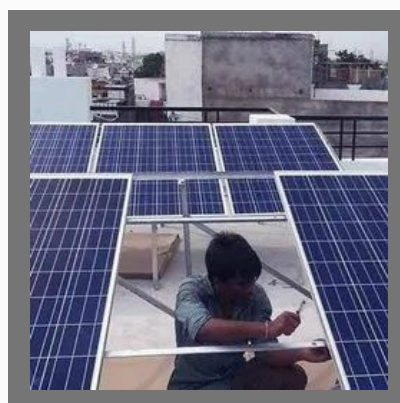
Solar Panel Installation
