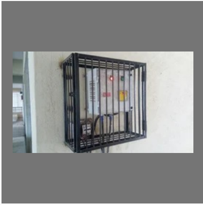
Safety Box Fabrication
