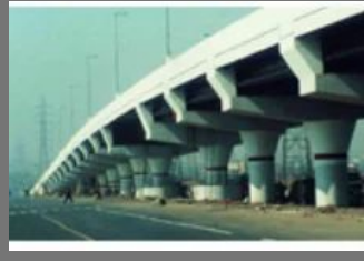
Flyovers Construction Service
