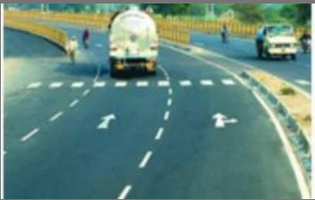
Roadways Construction Service
