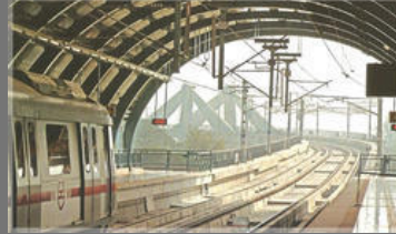
Elevated Viaducts For Delhi Metro Rail Corporation
