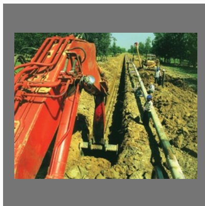
Saharanpur Pipeline Project
