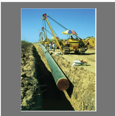
Dahei Uran Pipeline Project
