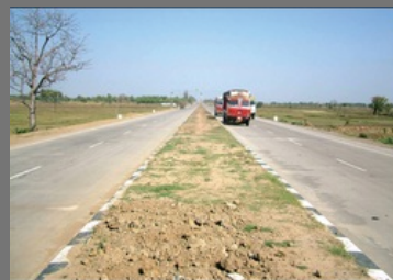
Shergati Highway Construction
