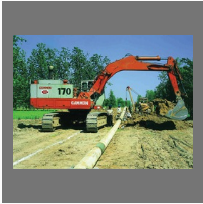
Barauni Patna Pipeline Project
