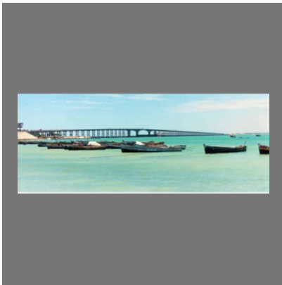
Pamban Bridge Construction
