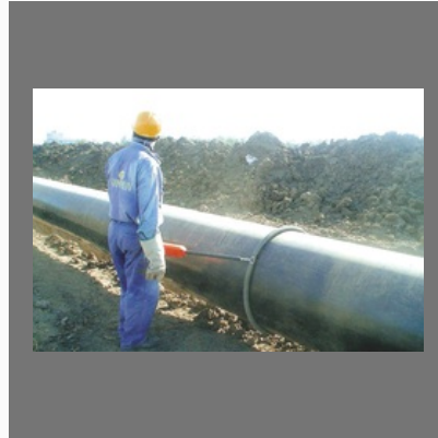
Mora Sajod Pipeline Project
