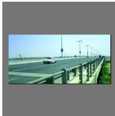
Delhi Noida Bridge Construction
