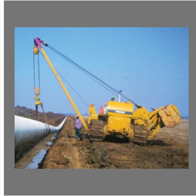
Paradip Pipeline Project
