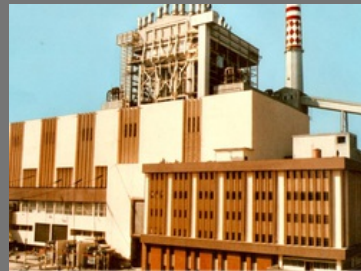
Thermal Power Station
