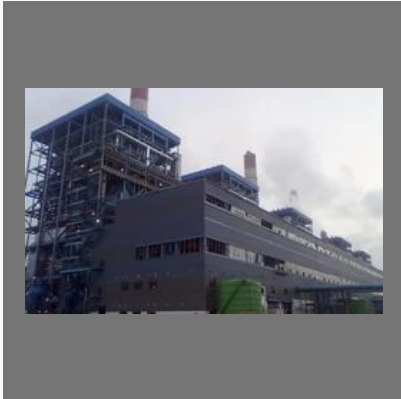
Power House Civil Engineering Projects
