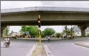
Bridges And Flyovers
