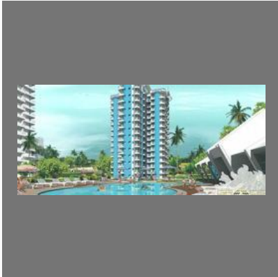
Hotel Construction Services
