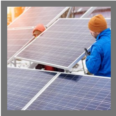
Solar Panel Installation Services
