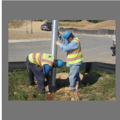
Street Light Installations Services
