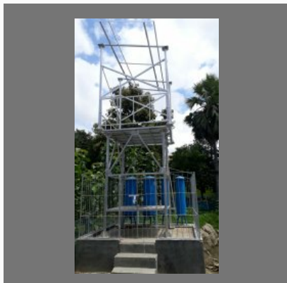
Arsenic Removal Plant
