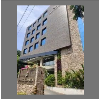
Commercial Construction Service
