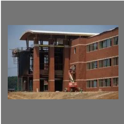
School Building Construction
