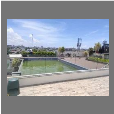
TERRACE SWIMMING POOL CONSTRUCTION
