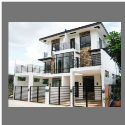
Residential House Construction Service
