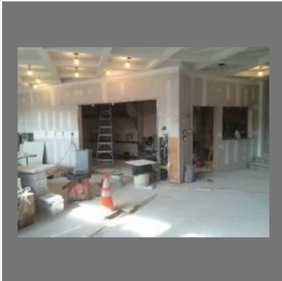
Restaurant Construction Service
