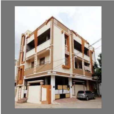
GBI Builders Apartment Construction
