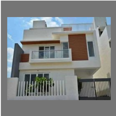
GBI Builders House Construction
