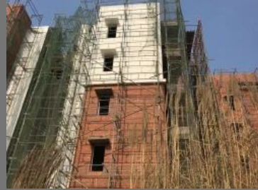
GBI Builders Civil Contractors
