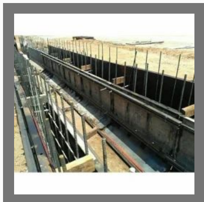
RCC DRAIN WORK CONTRACTORS
