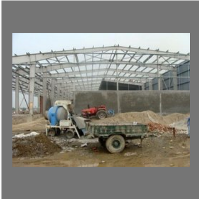
Pre Engineered Building
