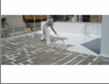
Terrace Water Proofing Services
