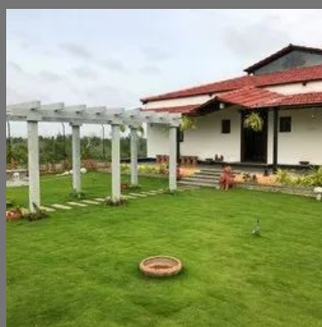
FARM HOUSE CONSTRUCTION
