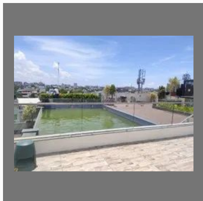
TERRACE SWIMMING POOL CONSTRUCTION
