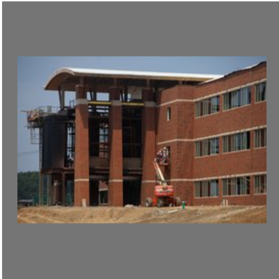
School Building Construction
