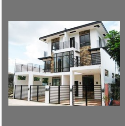
Residential House Construction
