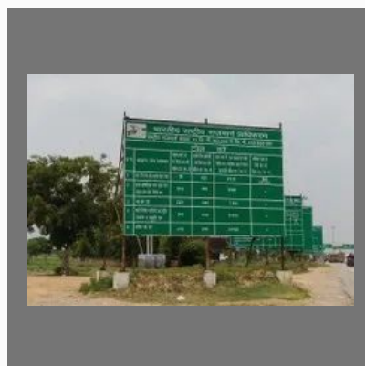
Cantilever Sign Boards
