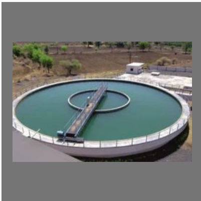
Process Water Treatment Plant
