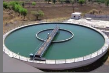
Sewage Treatment Plant with MBR
