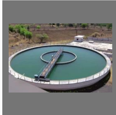
Compact Water Treatment Plant
