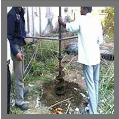
Earthing System Installation
