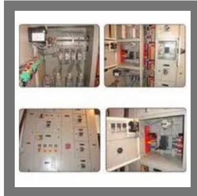
PCC & MCC Panel Installation
