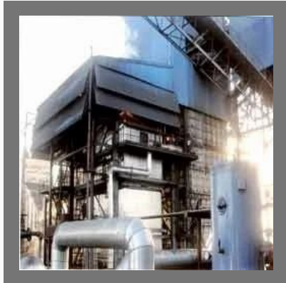
MS Pipeline Fabrication Service
