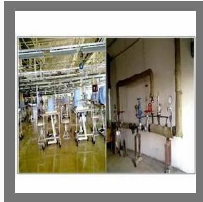
Steam Pipe Lines Fabrication Service
