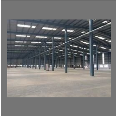
Shed Fabrication Service
