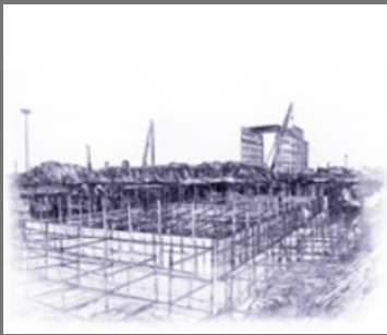
Power Building Construction Service
