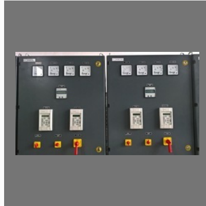
DG Synchronization Panel
