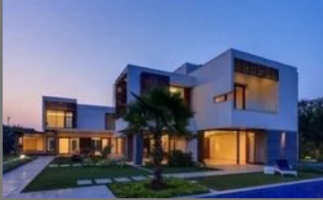
Civil Construction Service
