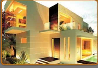
Industrial Building Construction
