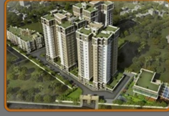
Residential Building Construction
