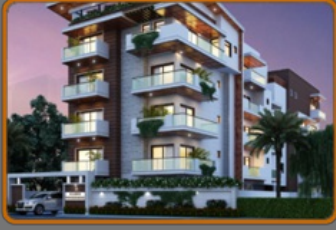
Commercial Building Construction Services
