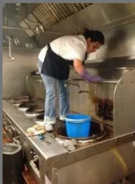
Kitchen Exhaust Deep Cleaning
