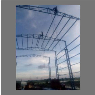
Warehouse Roofing Shed
