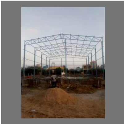
Badminton Court Construction Services
