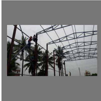
Warehouse Roofing Shed
