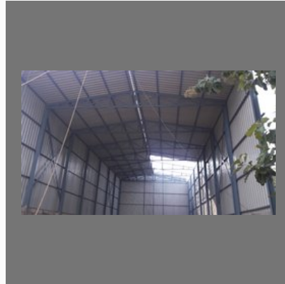
Residential Terrace Roofing Shed
