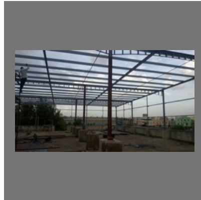
Marriage Hall Roofing Shed
