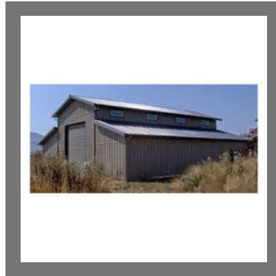
Godown Roofing Shed
