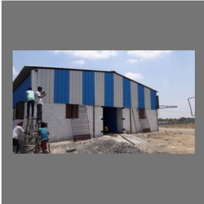
Roofing In Chennai
