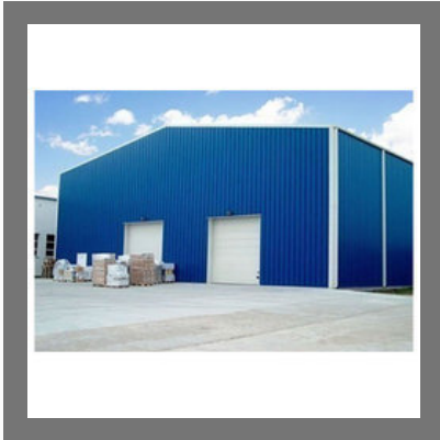
Factory Roofing Shed
