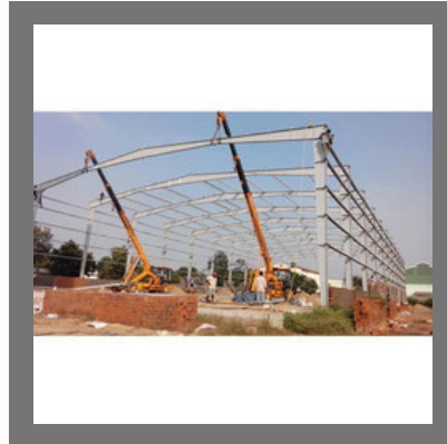
Industrial Steel Structure
