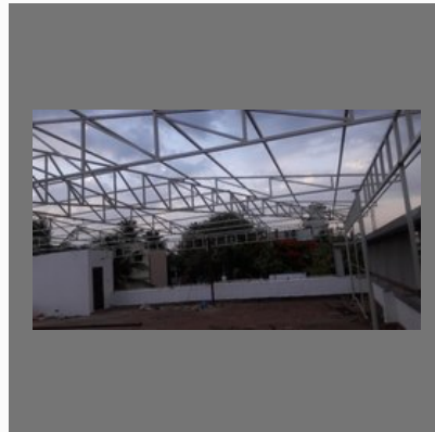
Roofing Service Shed in Chennai
