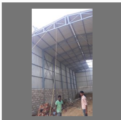
Warehouse Roofing Shed
