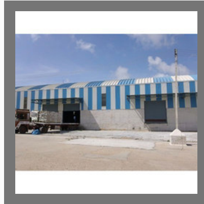
Industrial Godown Roofing Shed
