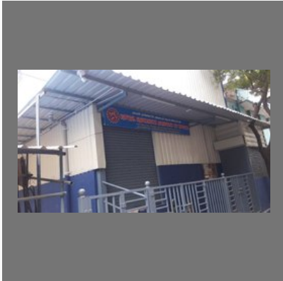
Factory Roofing Sheds
