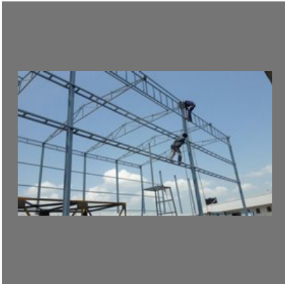
Factory Terrace Roofing Shed
