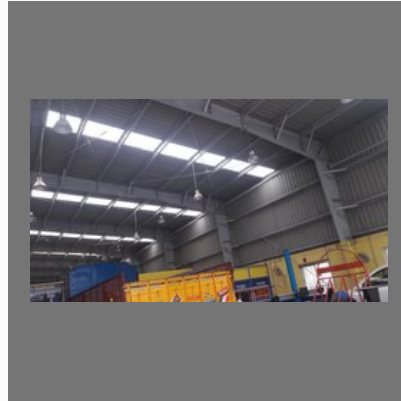
Metal Roofing Sheds Work
