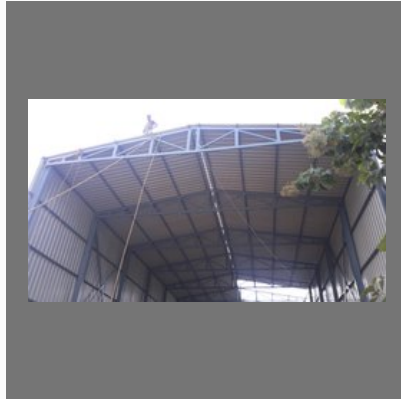
Temple Shed Roofing
