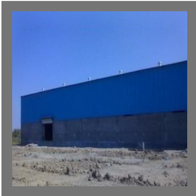
MS Prefabricated Roofing Shed steel
