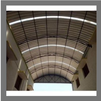
Terrace Arch Roofing
