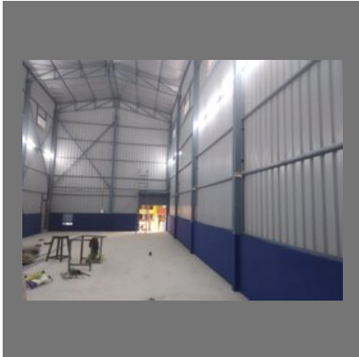
Badminton Court Construction Services
