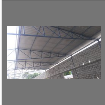
Steel Roofing Shed
