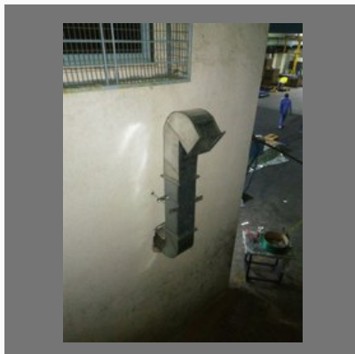
Ducting And Insulation Works
