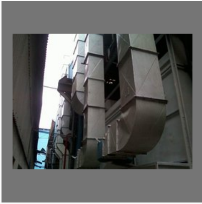
Industrial Ducting Works
