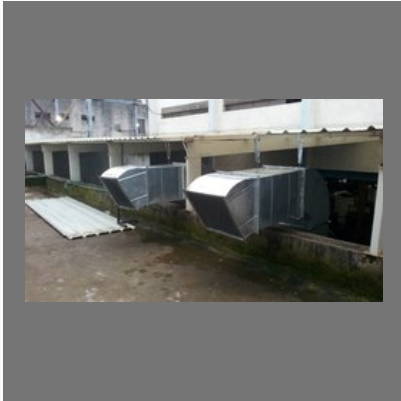
HVAC Ducting Work
