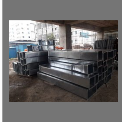
HVAC Ducting Work
