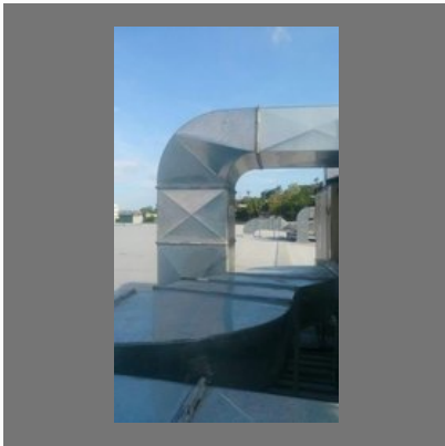
Industrial Ducting Works
