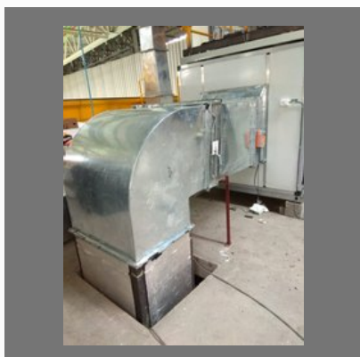
Stainless Steel Ducting Insulation Work
