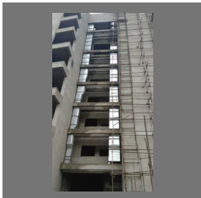
Duct Installation Services
