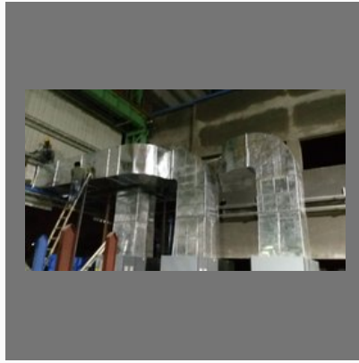
Industrial Ducting Works
