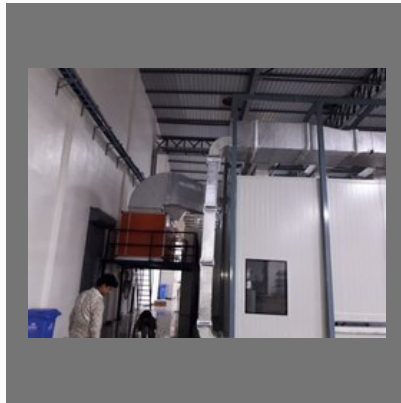
HVAC Ducting Work
