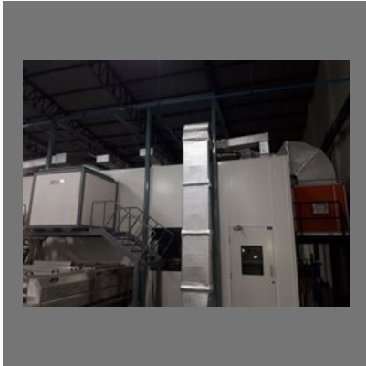
Duct Installation Services
