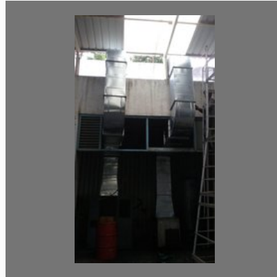
Duct Installation Services
