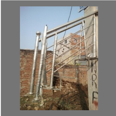
Steel Stairs Railing
