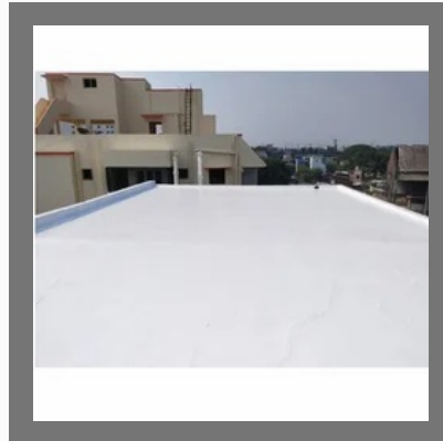
Terrace Water Proofing Services
