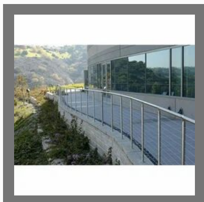
Stainless Steel Railing
