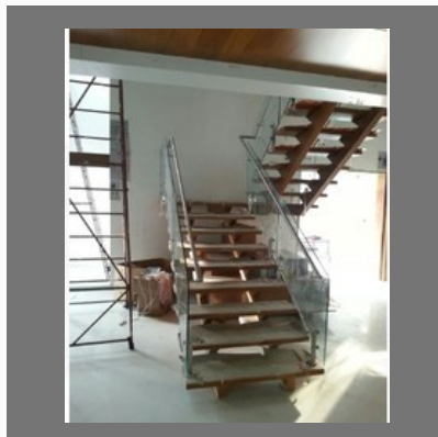
SS Stair Railing
