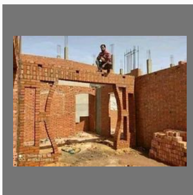
House Construction Services
