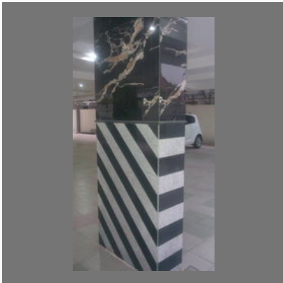
Granite Wall Fixing
