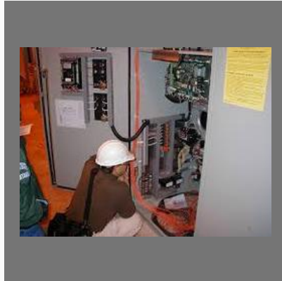
Control Panel Installation Service
