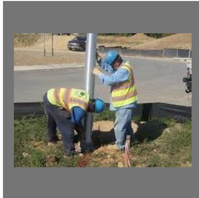
Street Light Pole Installation Service
