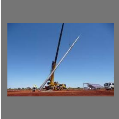
Street Light Pole Erection Service
