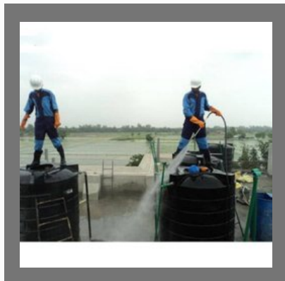
Commercial Water Tank Cleaning Service
